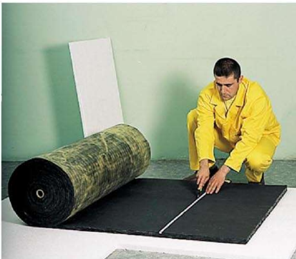
Cut to shape the Duct Liner.
