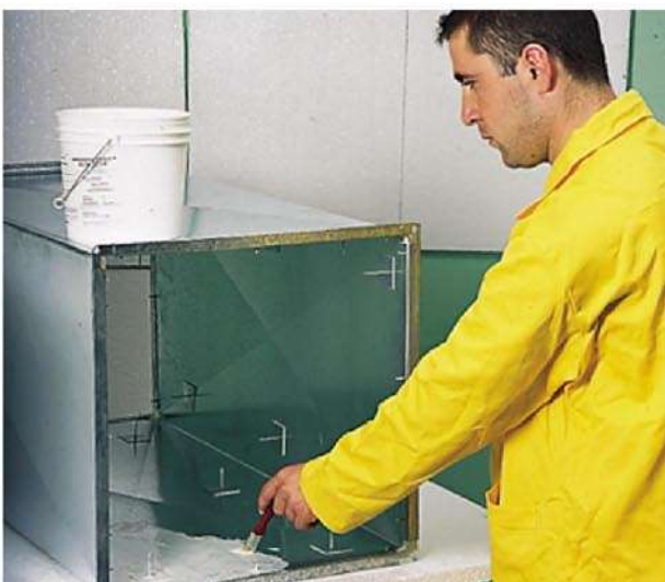
Apply suitable adhesive to duct surface before positioning Duct Liner over mechanical fastener pins.
