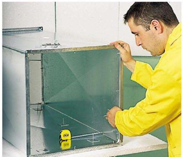
Affix mechanical fastener pins in accordance with manufacturers instructions.
