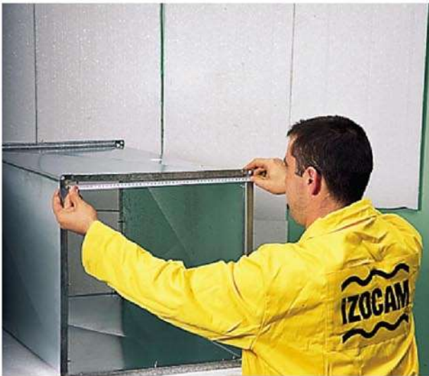
Measure the dimensions of the duct.
