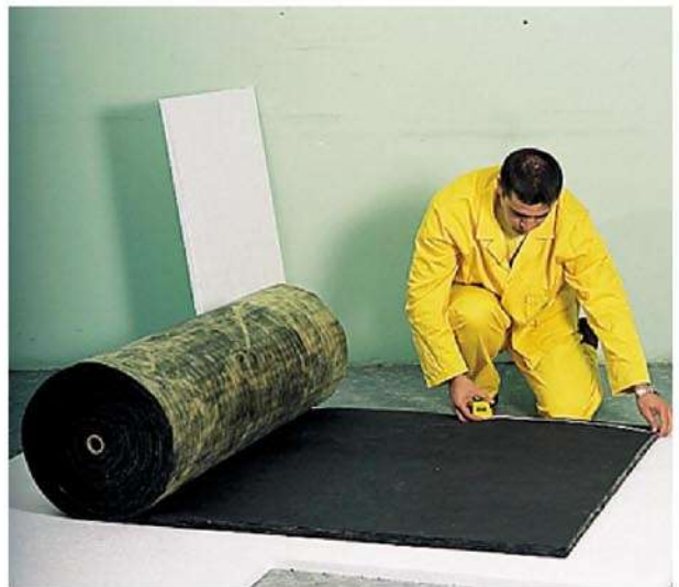
Do the marking in accordance with measured dimensions on the Duct Liner.
